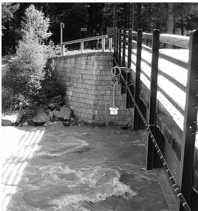
FIG. 5 - Ponte Maria hydrometric station (1100 m a.s.l.), with the staff gauge on the right bank of the bridge and the ultrasonic hydrometer in the centre.
